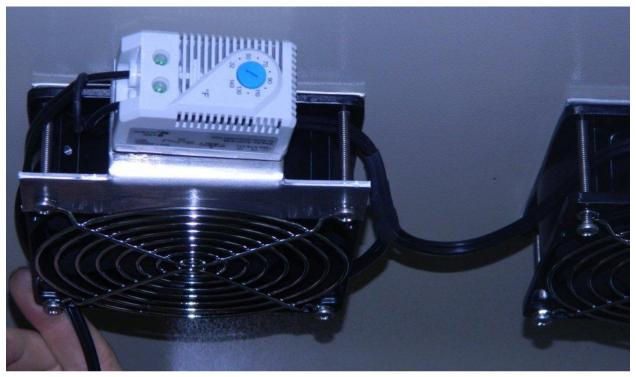
Place thermostat onto thermostat bracket
