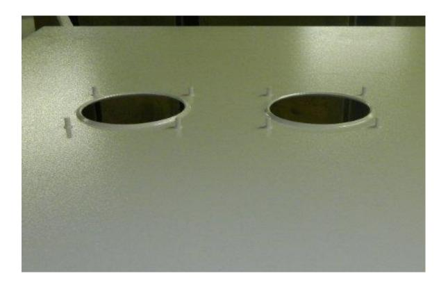
Top view of enclosure with Alumishield removed showing fan hole cut outs
