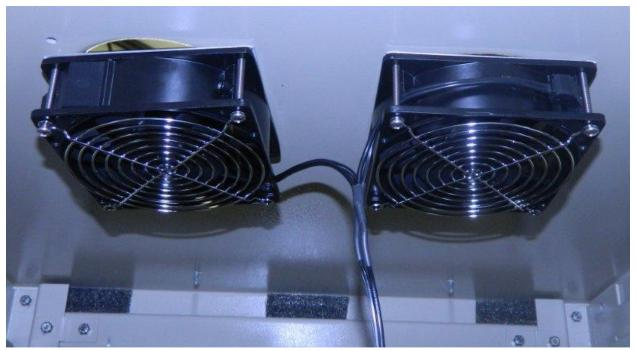
Place the fan finger guard under fan (NOTE: fan wire screen is above fan) and insert fourth screw into roof of the enclosure
