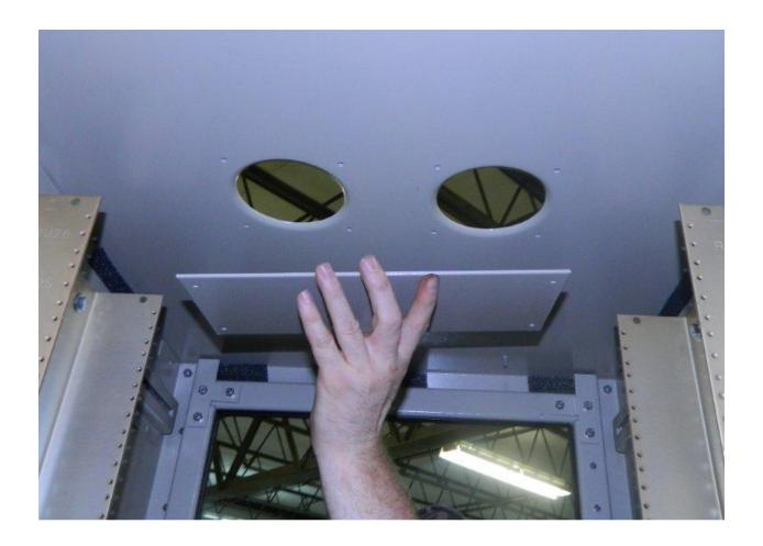
Under the cover plate there are two prepunched fan cut-outs with tapped holes for screws.
