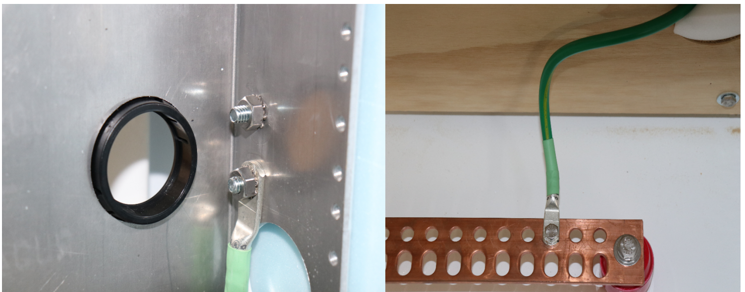
FIGURE 13: SINGLE LUG GROUNDING FOR RAILS
