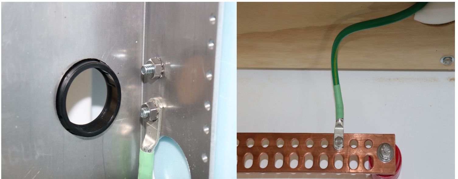
FIGURE 13: SINGLE LUG GROUNDING FOR RAILS
