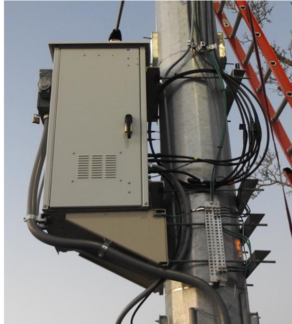
Figure 2: Typical pole installation shows an area roughly four (4) inches wide in the middle of the PMS in contact with the pole.
